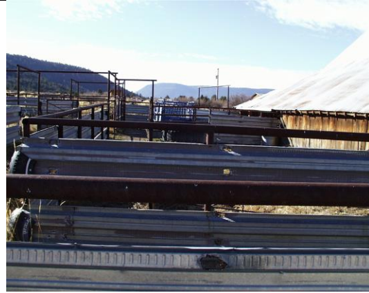
11. Corrals, pipe with metal sides
